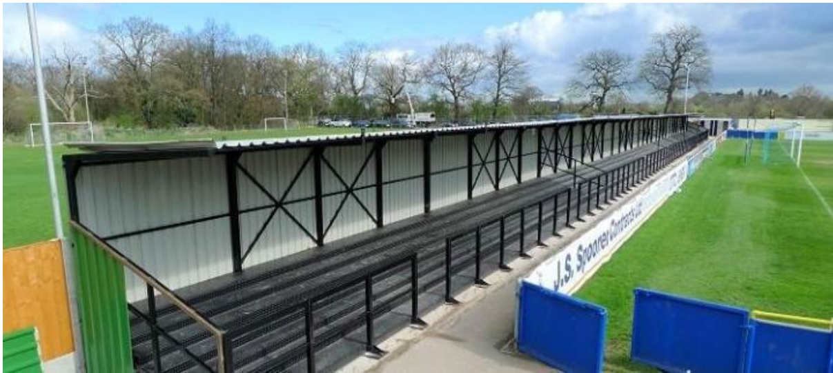
Drain Tech End
