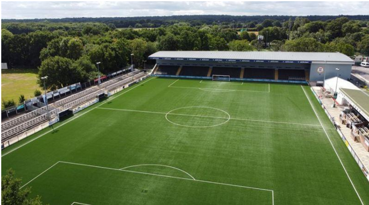
The new Enclosure
